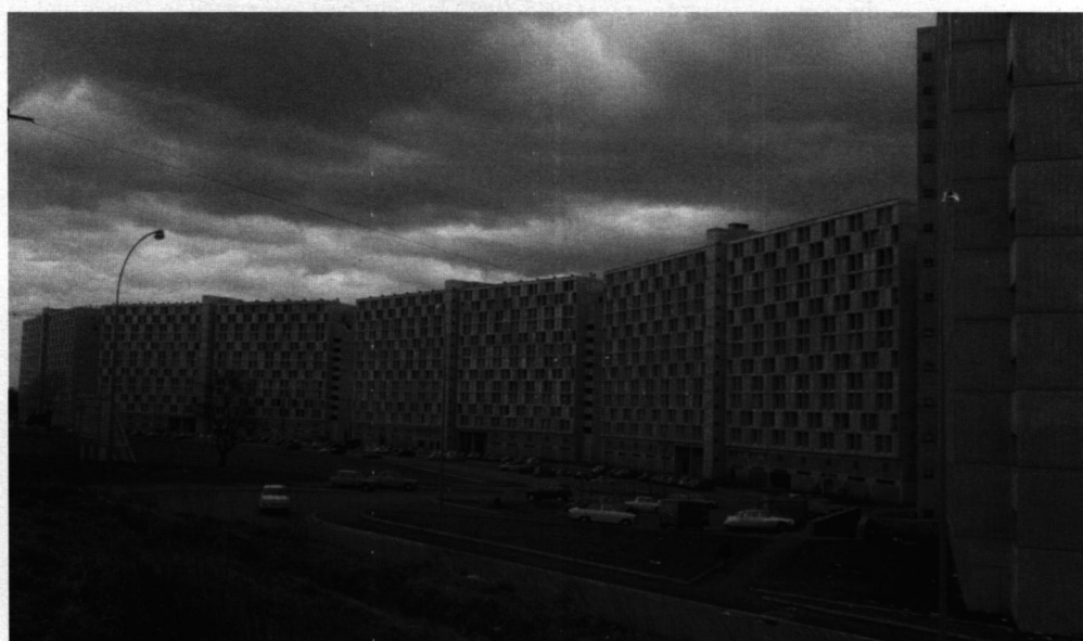
Figures 4 and 5. The residential blocks of the ZUP in Sainte-Croix, Bayonne, in their final phase of construction. Source: Musée Basque et de l'Histoire de Bayonne (Photographs by Robert Hourgras).
